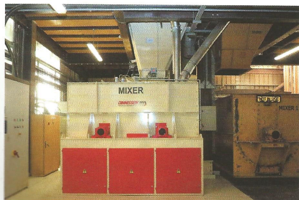
Left: The latest and biggest high-performance raw materials mixer unit installed in the mill. The older, smaller unit can be seen on the right
